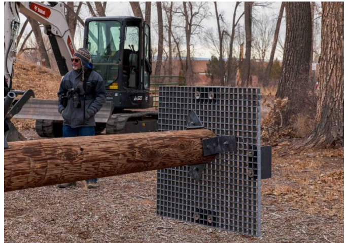
A closeup view of the platform installed atop the pole.
